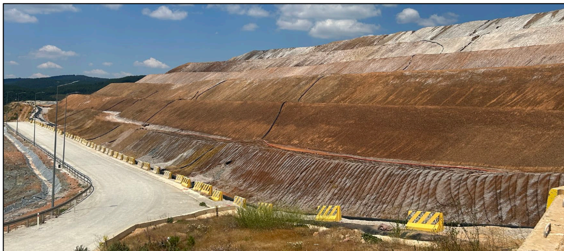
Figure 2-6: View of South Flank of HLF, showing residual leaching of bottom lift (Date: July 2026)
