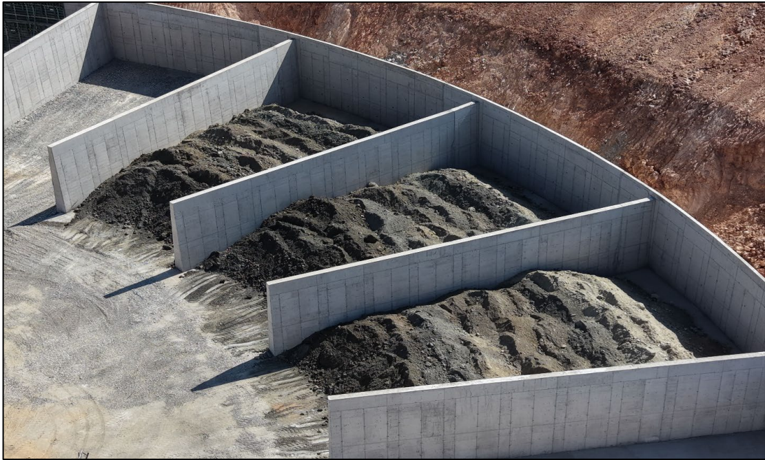
Figure 10-2: View of the four (or ten) ore bins with ore noting that the truck tipping area to the rear will be completed once forestry permits are received
