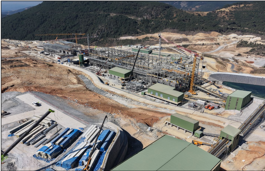
Figure 10-1: View of the plant (looking southwest) noting the completion status of the front end, contact water pond, ongoing construction work (note cladding planned to be applied post commissioning)
