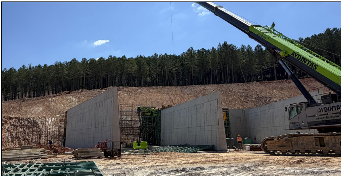
Figure 9-2: RoM Bin construction showing Bay no. 2 and 3 (the bays to the right are already completed)
