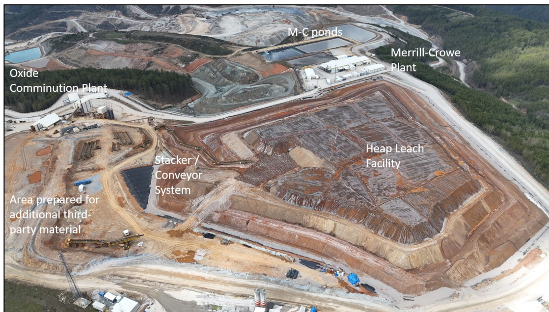
Figure 2-5: Aerial View of Phase 1 Oxide Project Heap Leach Facility and Associated Infrastructure, looking South (source: ACG; Date: April 2026)
