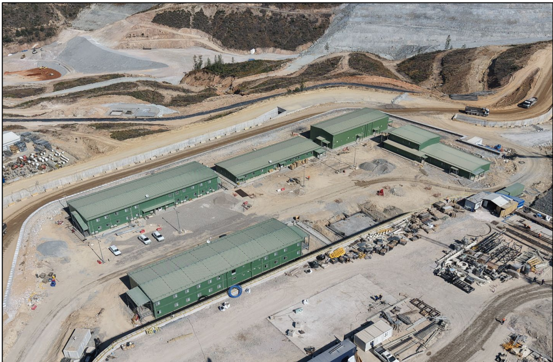
Figure 10-3: View of the administration area which is materially complete barring the ERT building (the concrete base can be seen)
