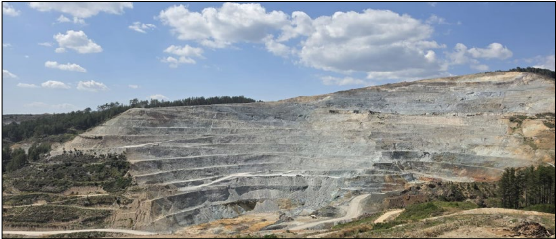
Figure 5-1: North Pit, looking NW (July 2026)
