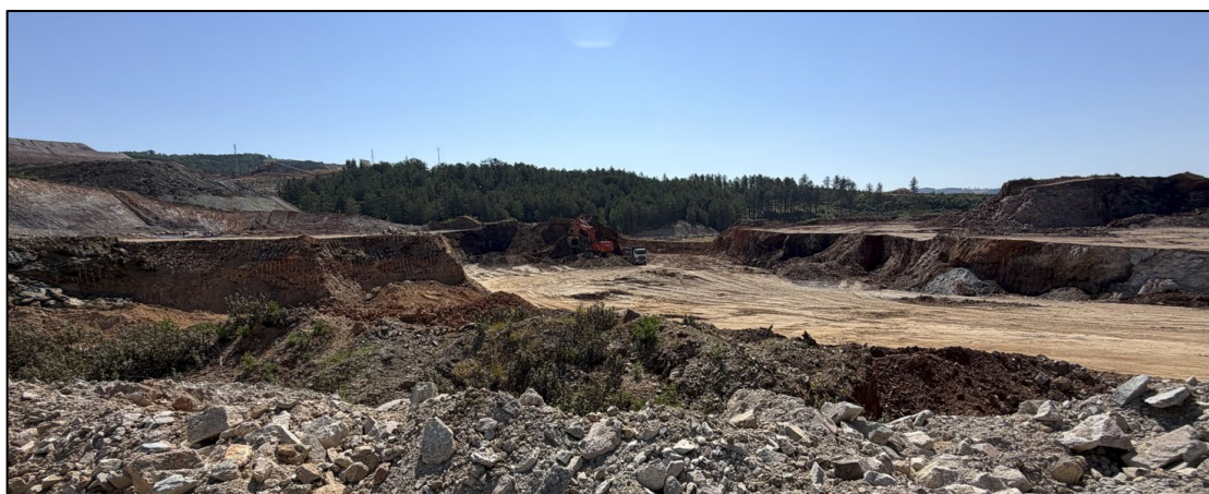
Figure 10-4: Bulk earthworks (oxide heap leach in the distance to the left)
