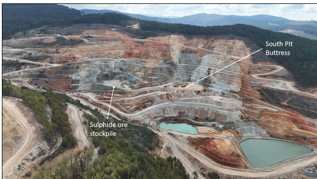
Figure 2-8: South and Central Pits, looking East (Date: July 2026)
