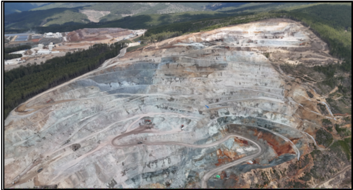
Figure 2-9: Pre-stripping at North Pit, looking northwest (Source ACG; Date: April 2026)
