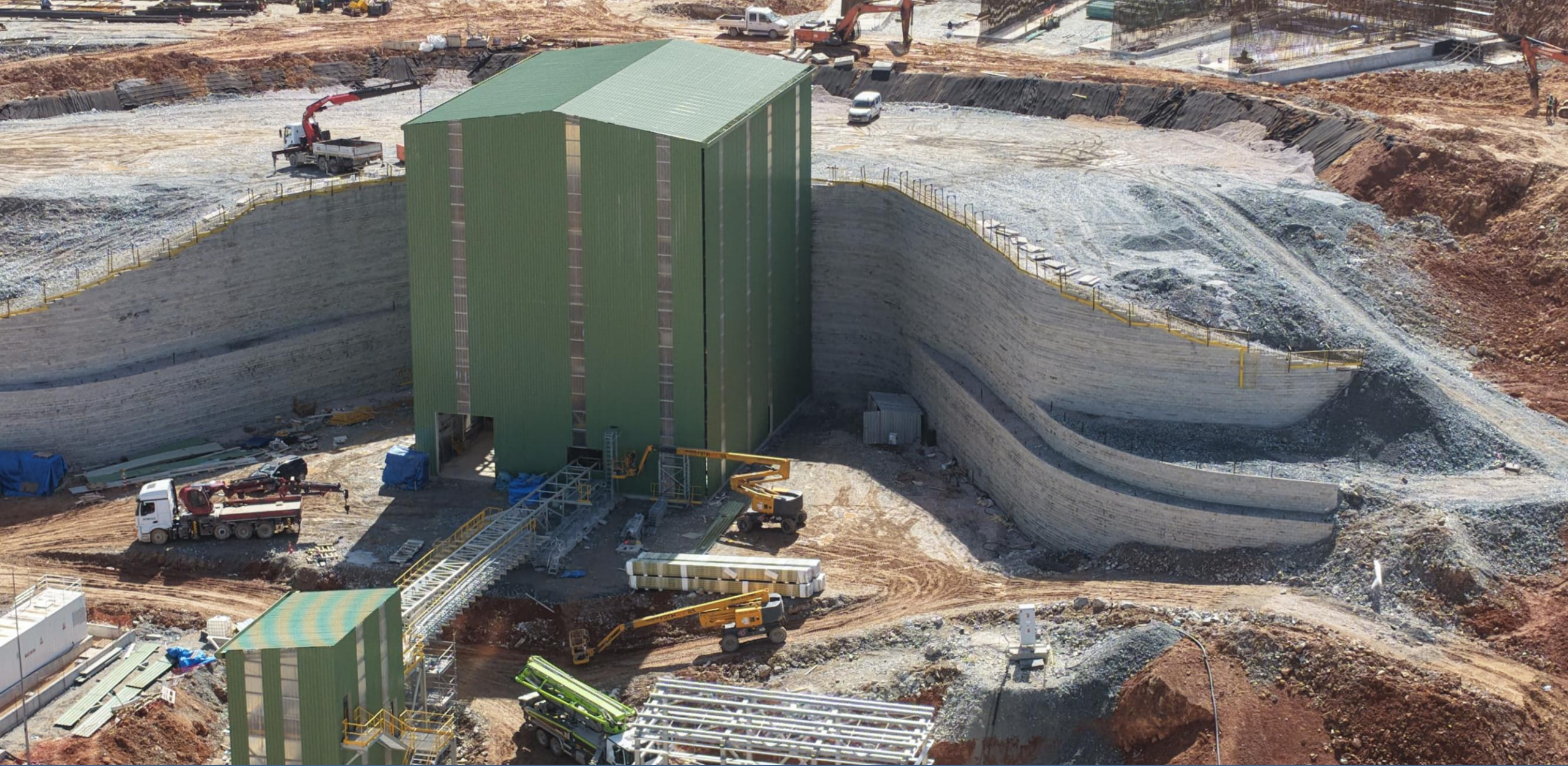
Primary crusher building and transfer tower
