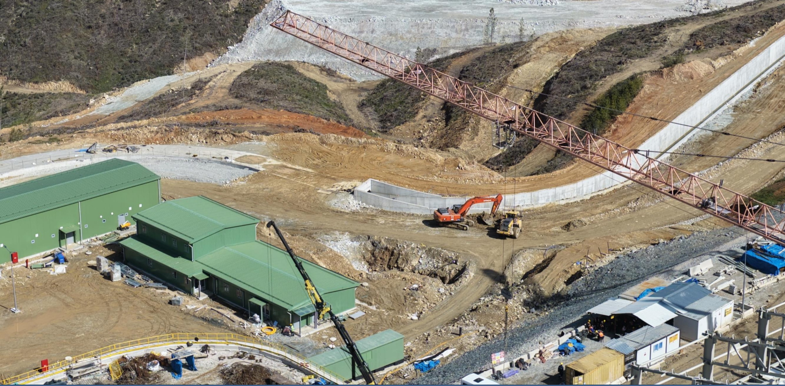
Saddle Dam administration area and diversion drain
