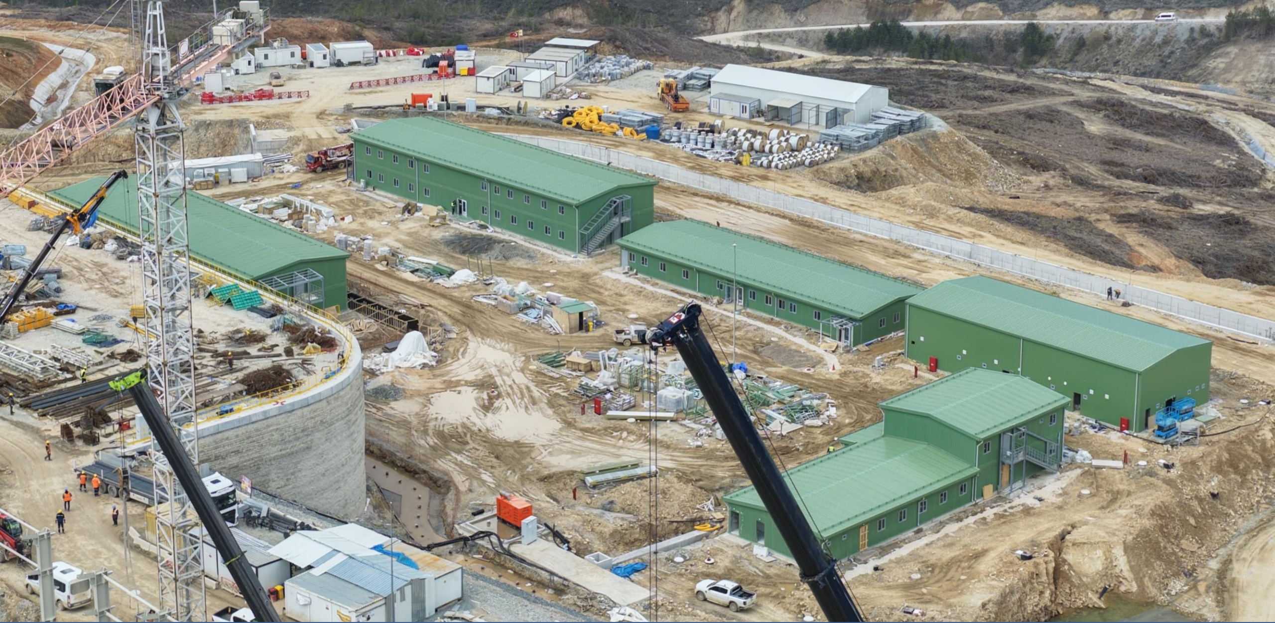
Administration area buildings nearing completion
