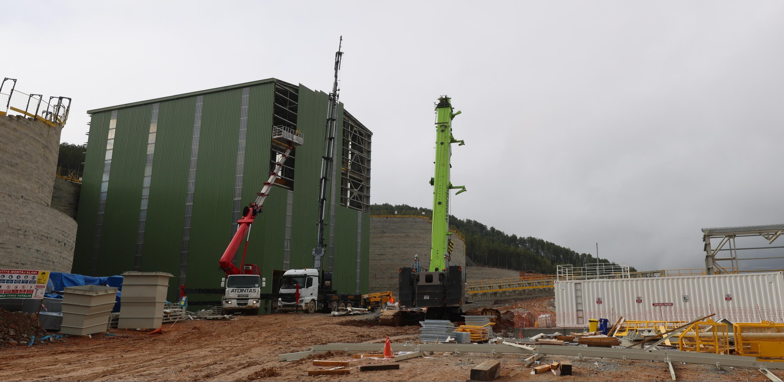
Cladding works progressing on the primary crusher building
