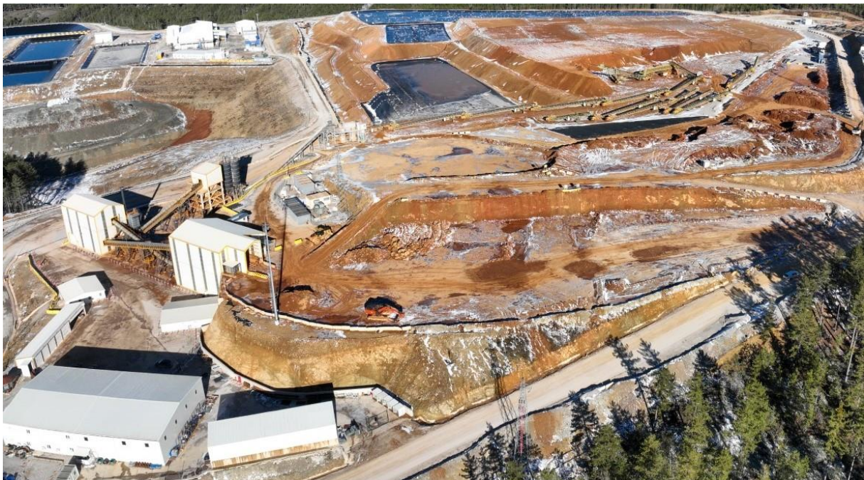
Figure 17.1 Oxide Project ore processing operations
