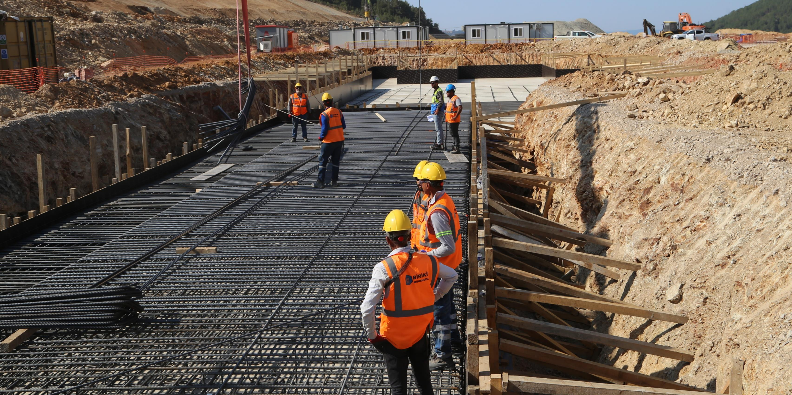
Rebar Workers on Fine Ore Bin Foundations
