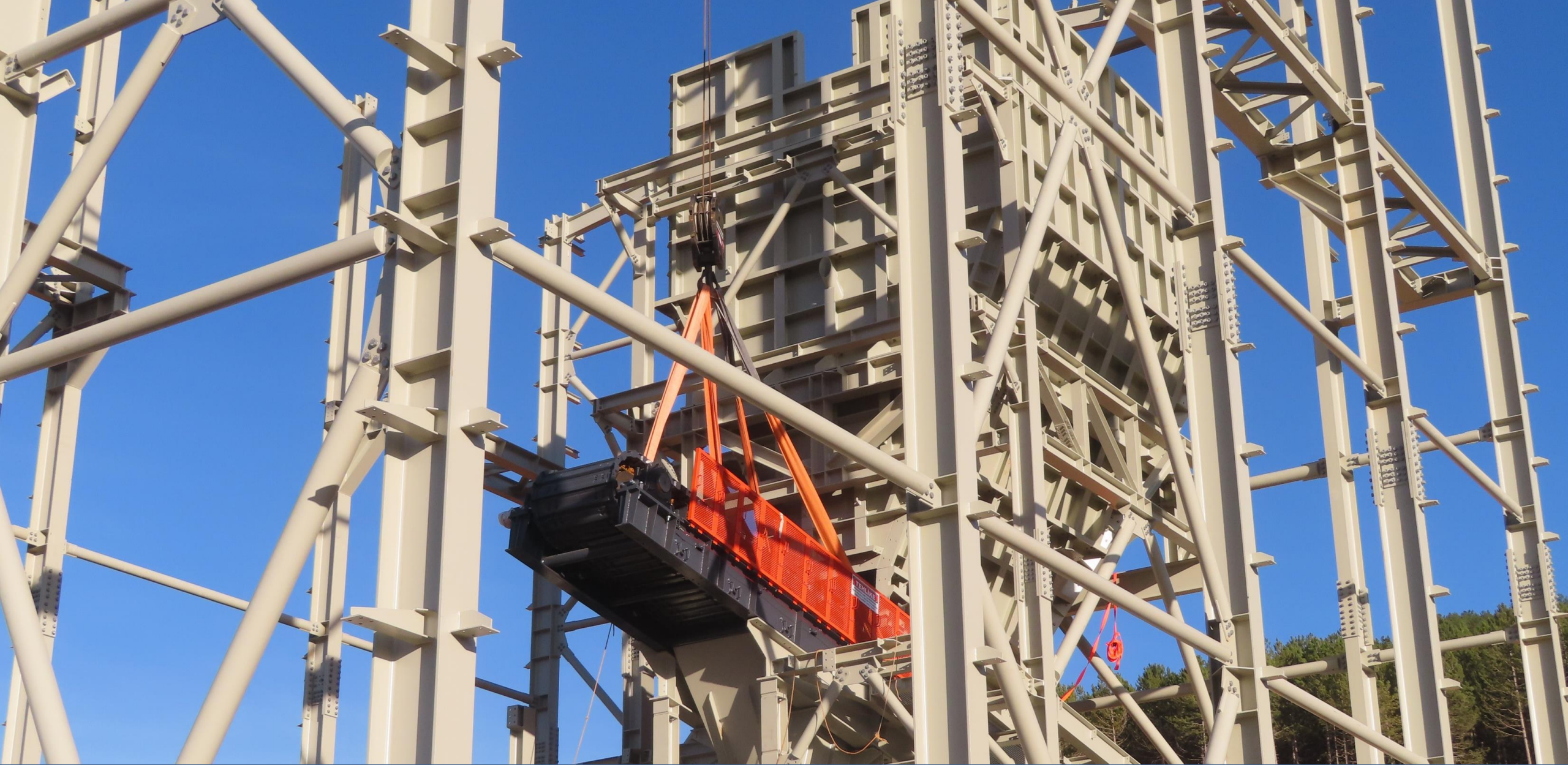
Apron Feeder Being Installed at Primary Crusher
