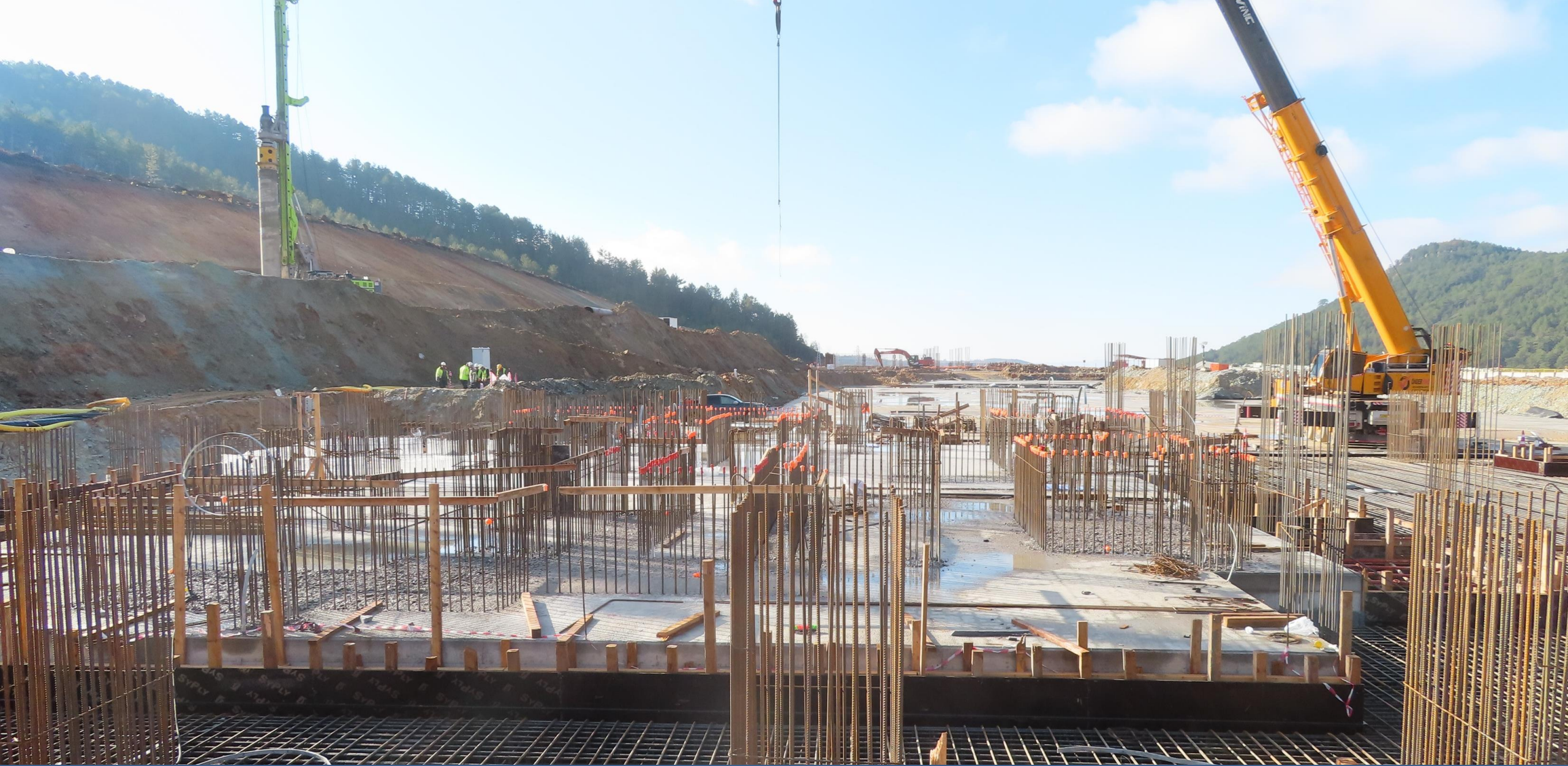
SAG and Ball Mills Foundation Slab Rebar Installation
