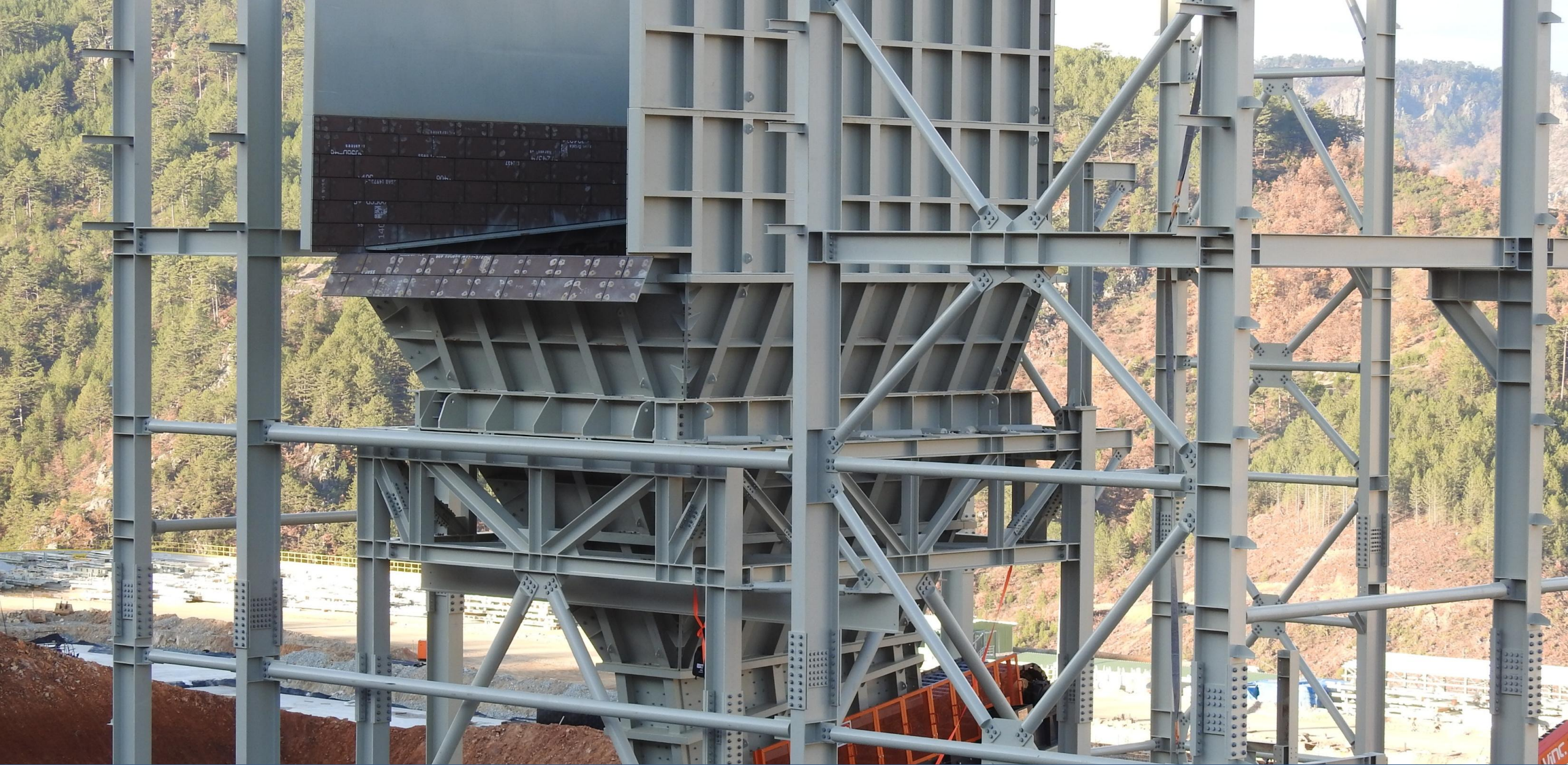
Primary Crusher Building ROM Bin Plate Feeder
