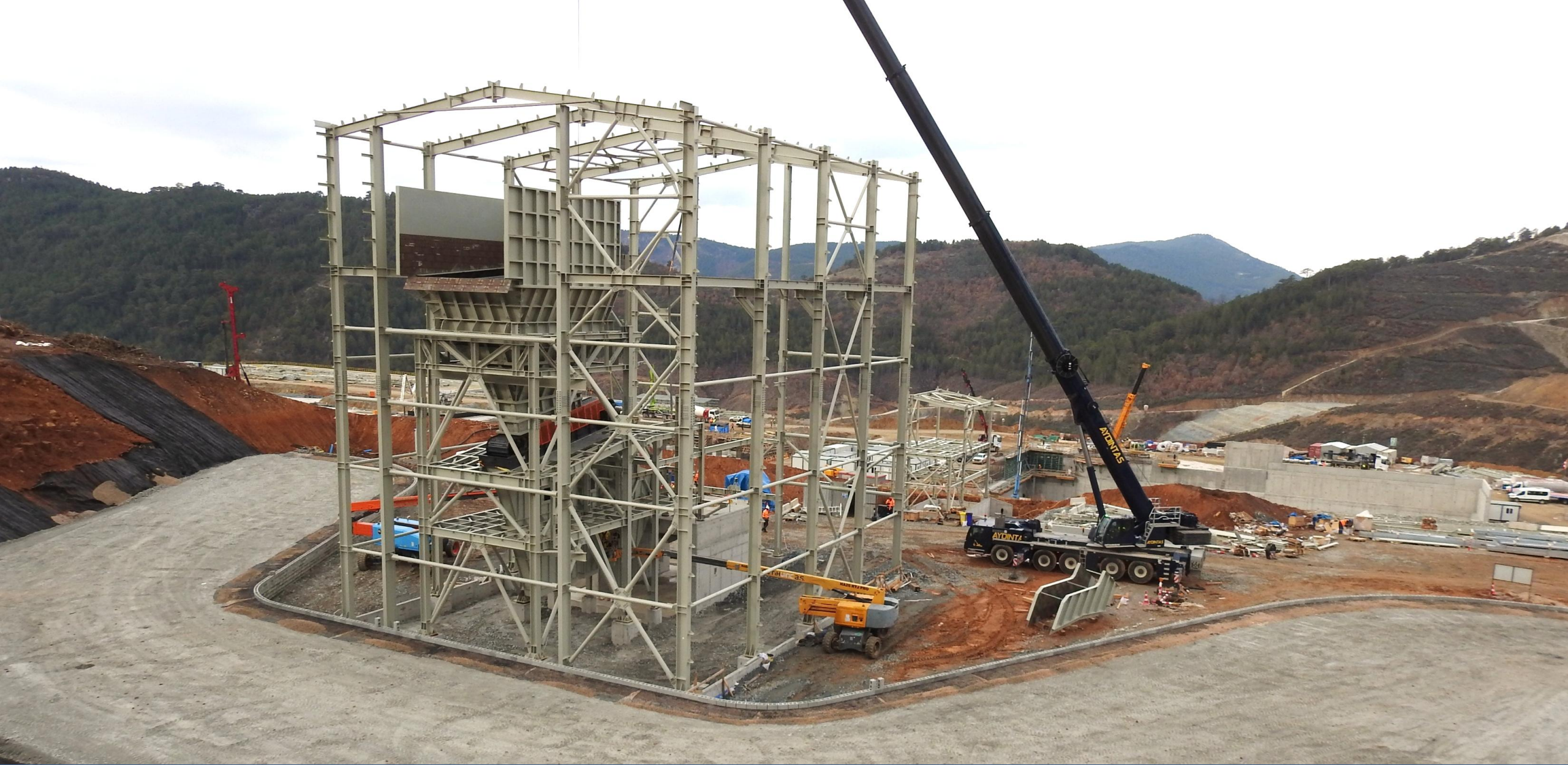
Primary Crusher Building With MSE Wall Construction
