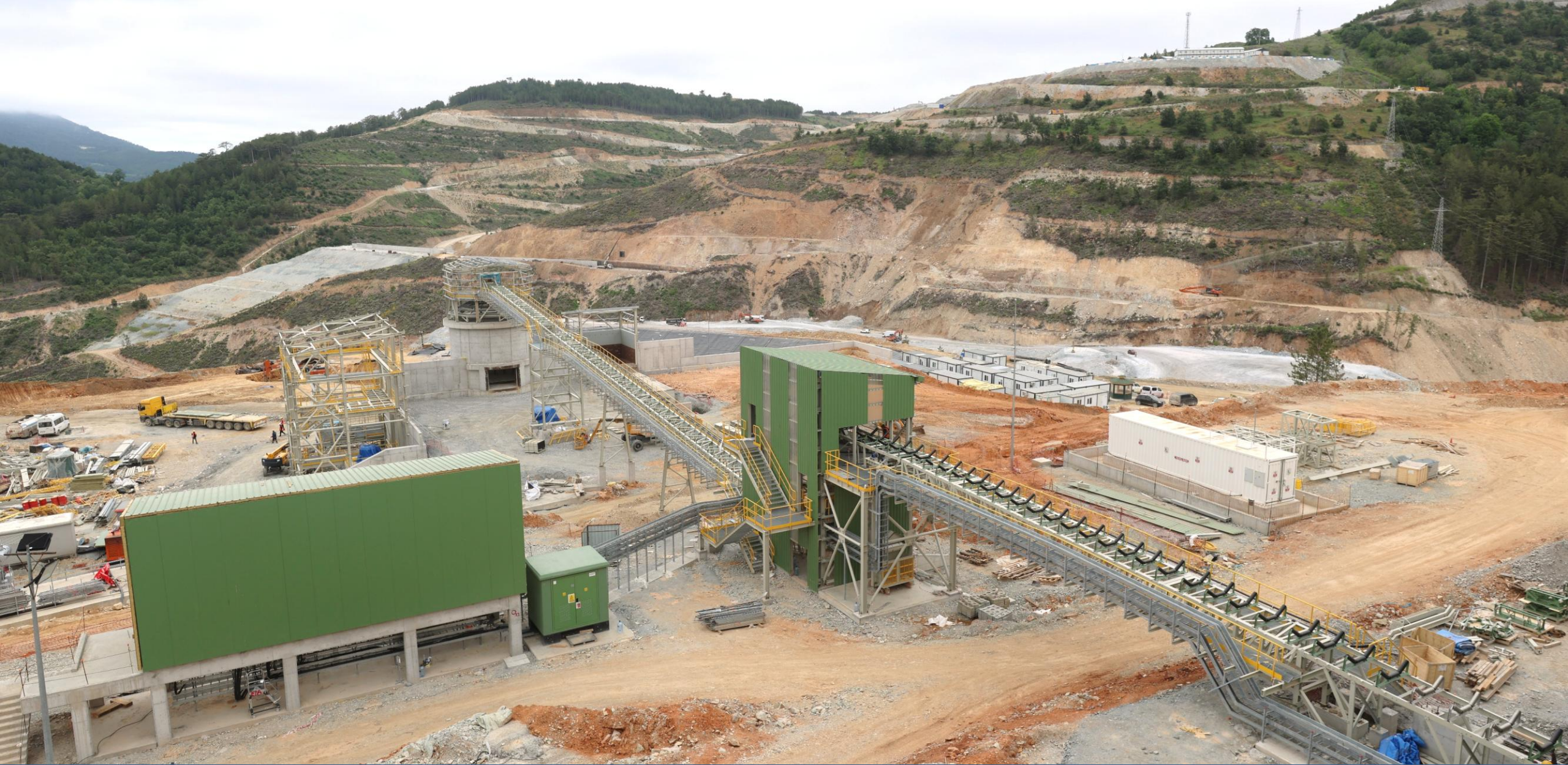
Grinding circuit conveyor system integrated into the processing plant, linking the primary crusher and mills
