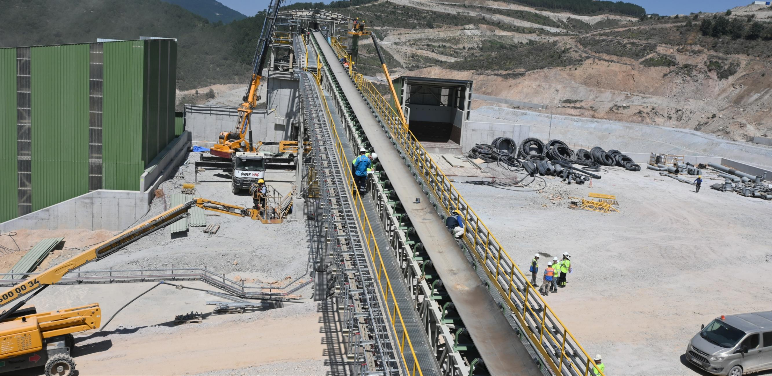
Main feed conveyor primary brusher to ore bin
