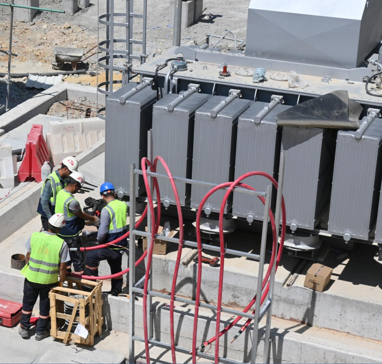
Main feed transformer and electrical feed line
