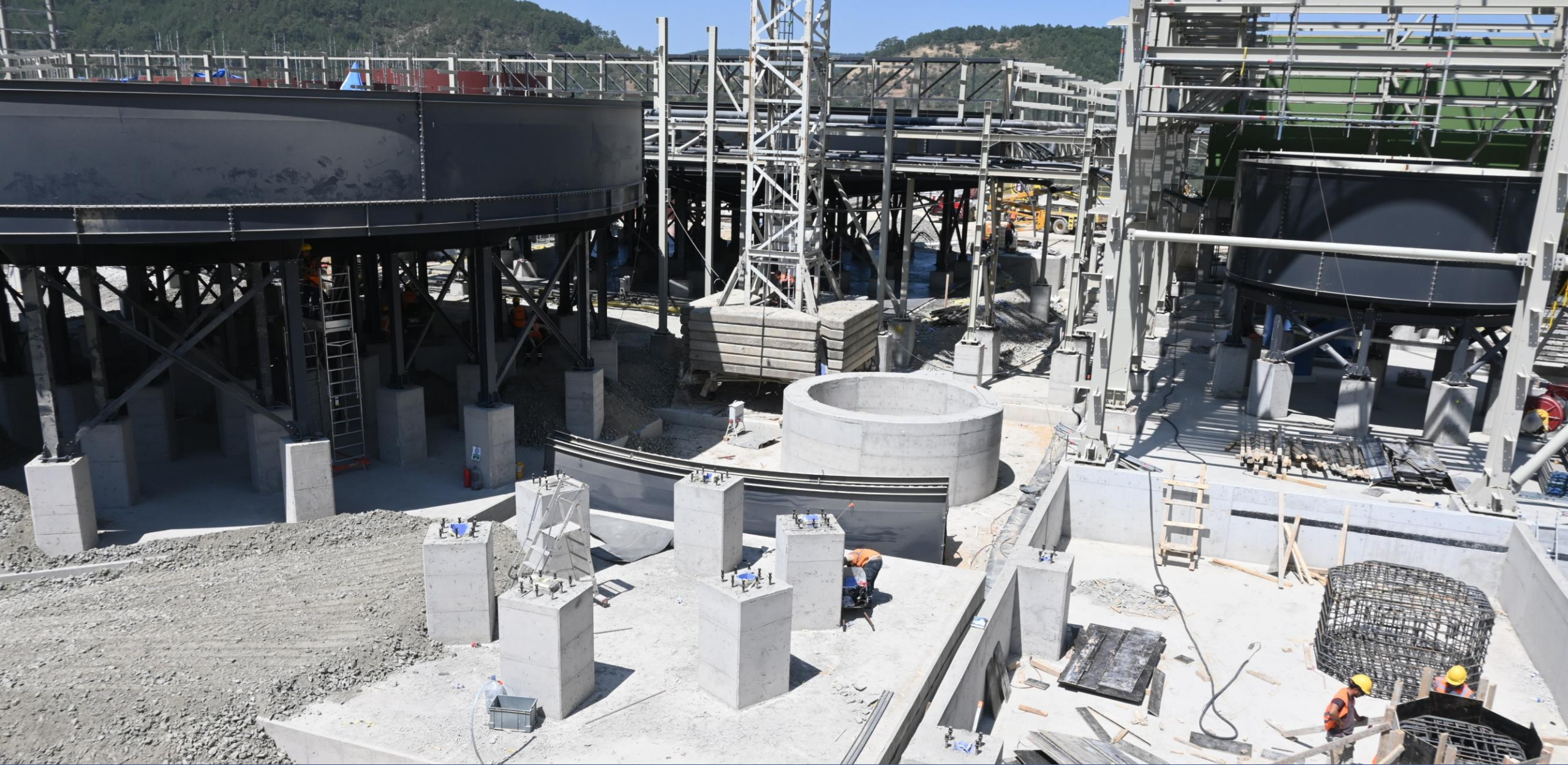
Lime silo and foundations works
